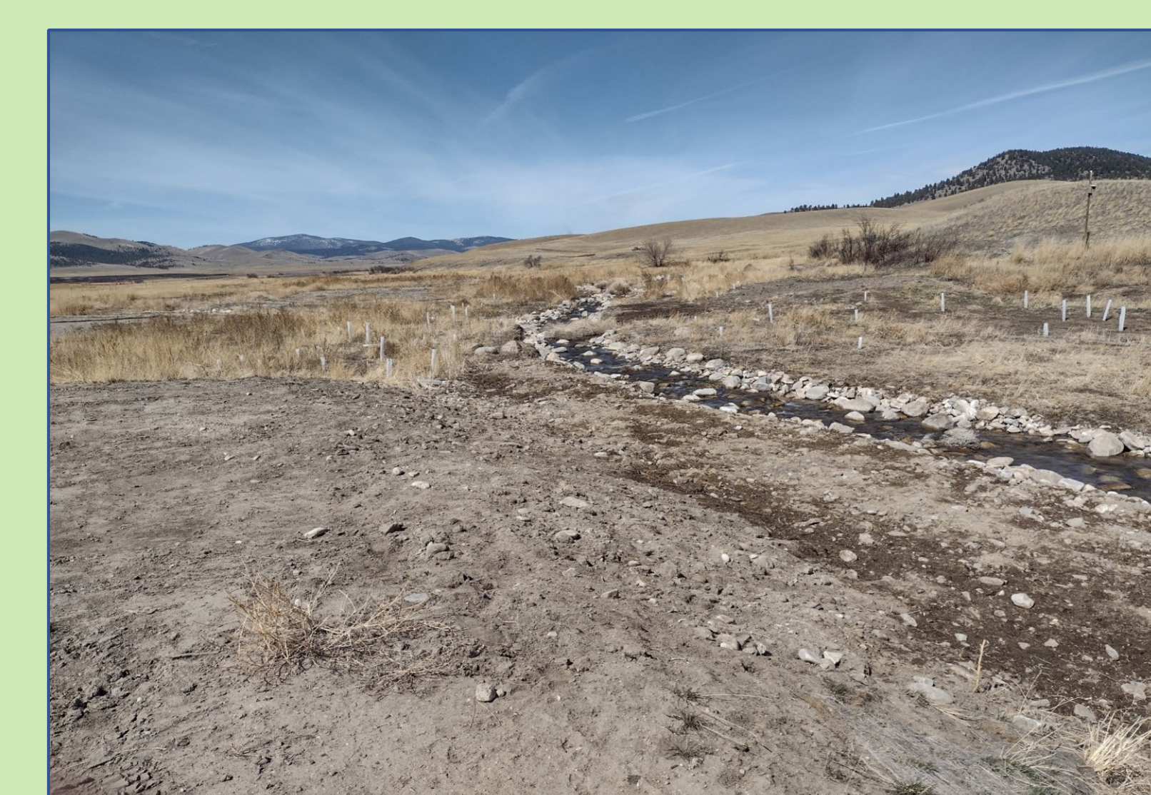
Figure 4. Stream channel profile after the restoration 'repair' and regrading work completed in spring 2022 (below).
